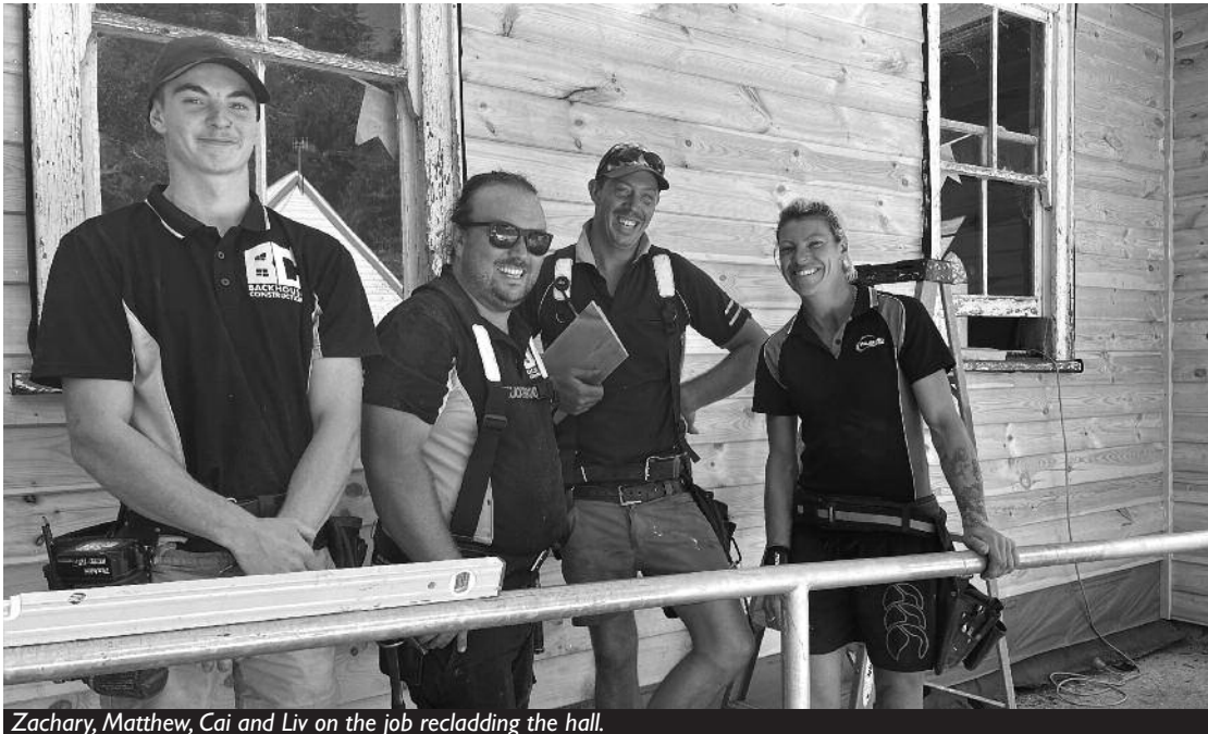
Zachary, Matthew, Cai and Liv on the job recladding the hall.
